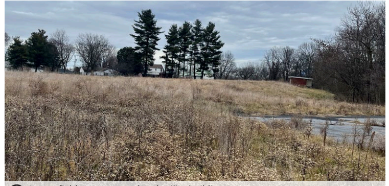
(D) Lower field, concrete pad and utility building.
