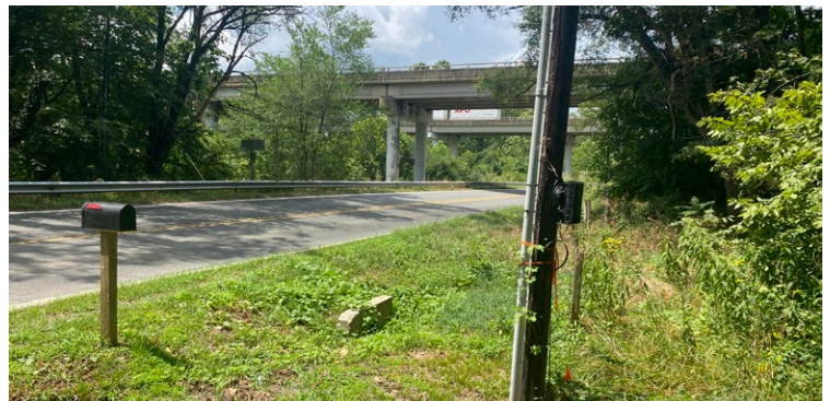
(F) View toward the I-81 underpass from the private driveway at 370 Bryce Blvd. Note: the culvert structure conveys water from Baker Parcel across Bryce Blvd.
