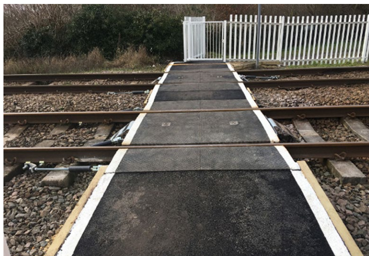
Pedestrian railroad crossing
