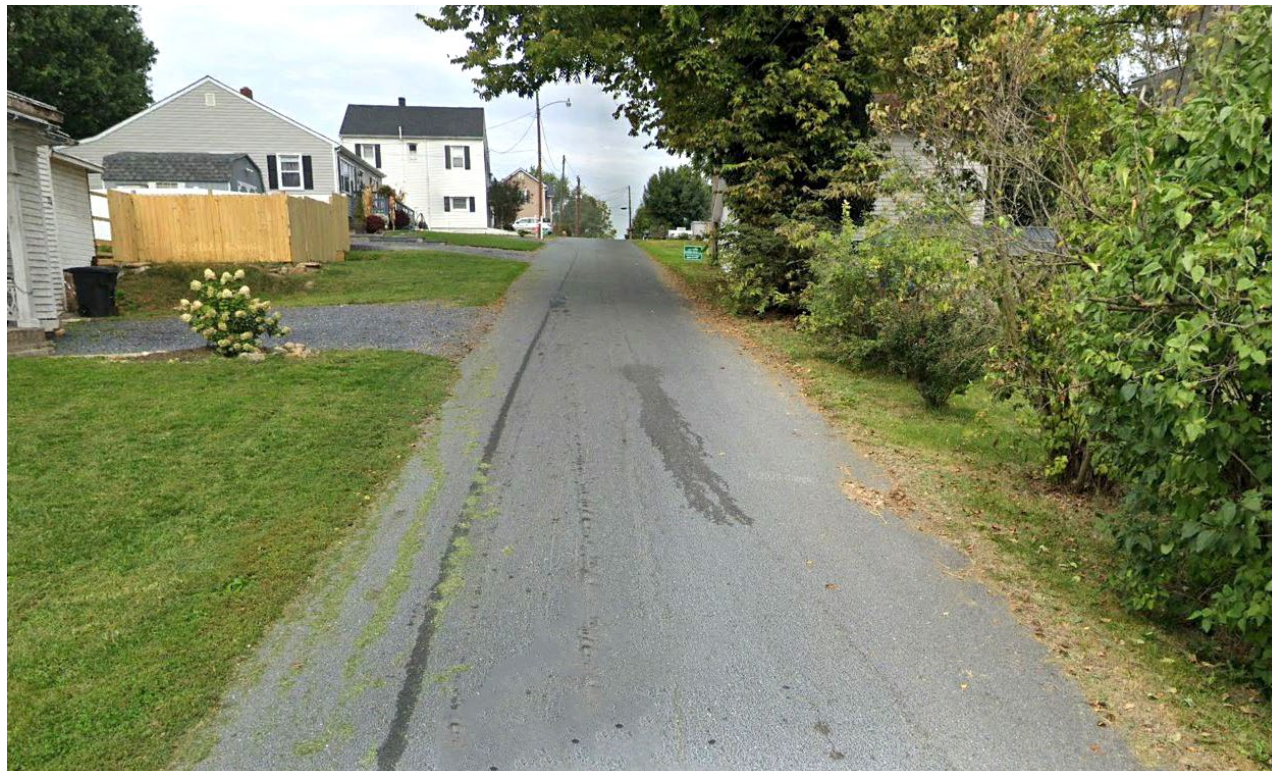
Existing Condition: Lower Wunder Street
