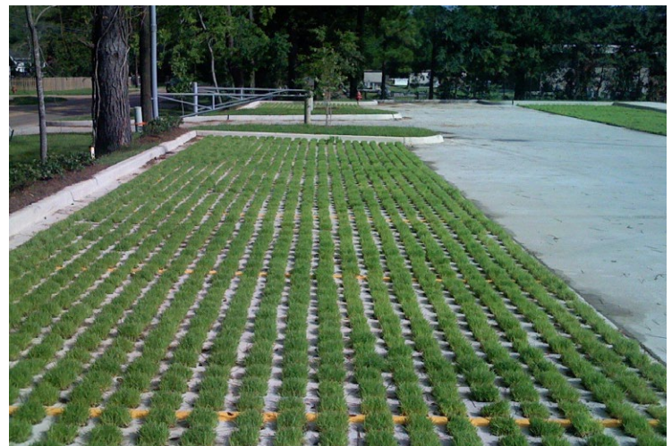
Renovated parking lot with permeable pavers
