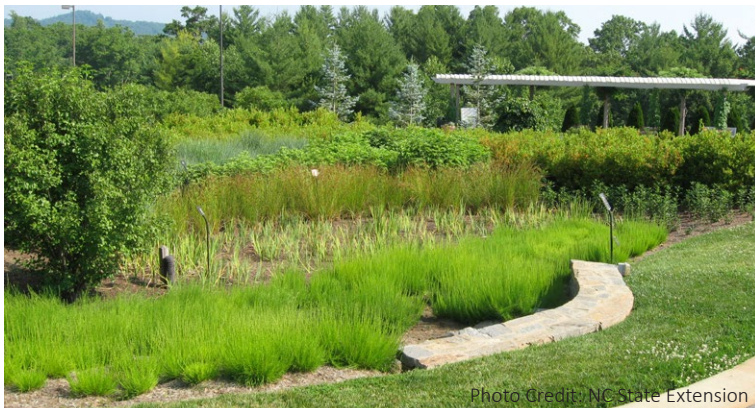
Stormwater management bioretention with native plants.
